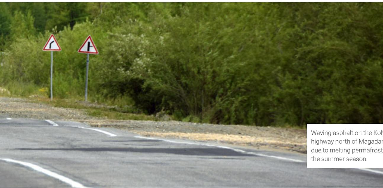
Waving asphalt on the Kolyma highway north of Magadan. This is due to melting permafrost during the summer season
