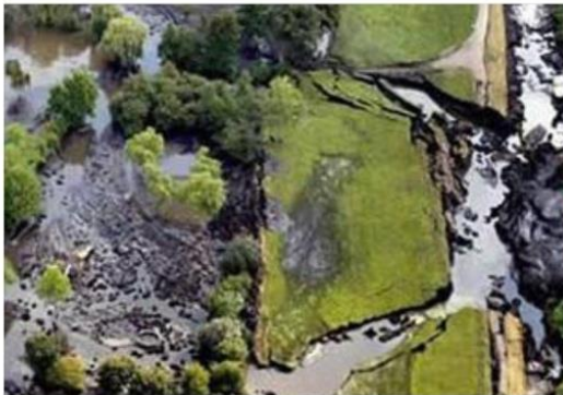
Levee breakthrough (drought)
