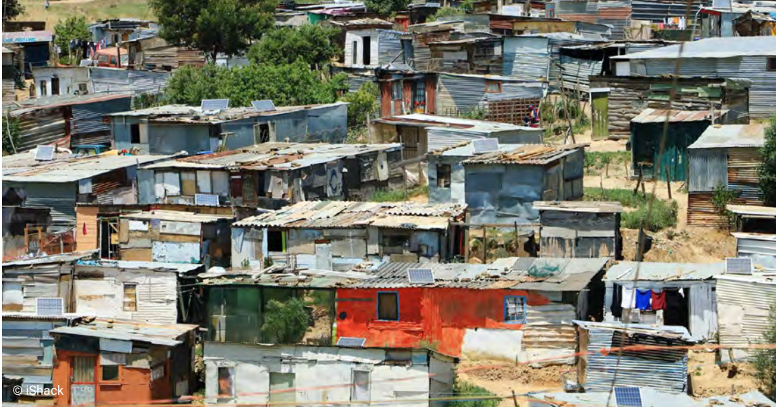
Installed solar panels over shacks and homes in South Africa.
