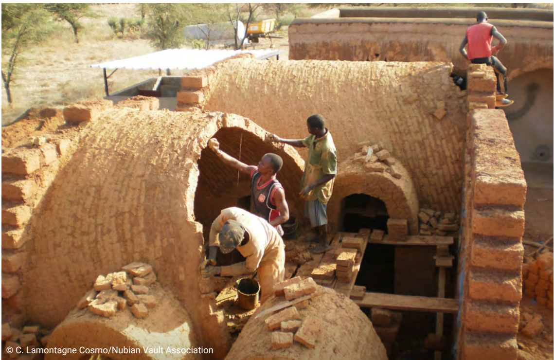
Four men working on the construction of a Nubian vault.
