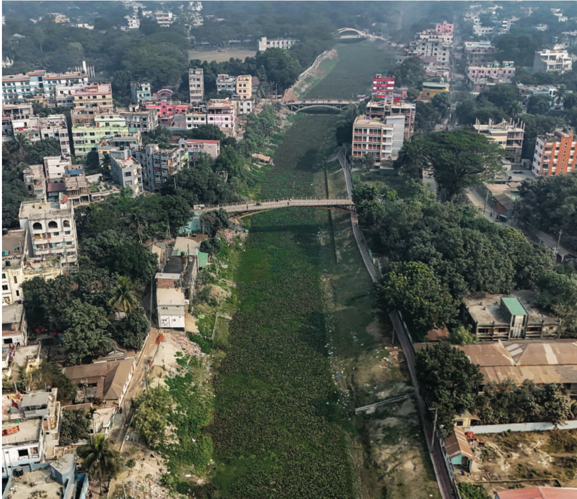
Photo 72: A view of Katakhlī Khal, Sirajganj
