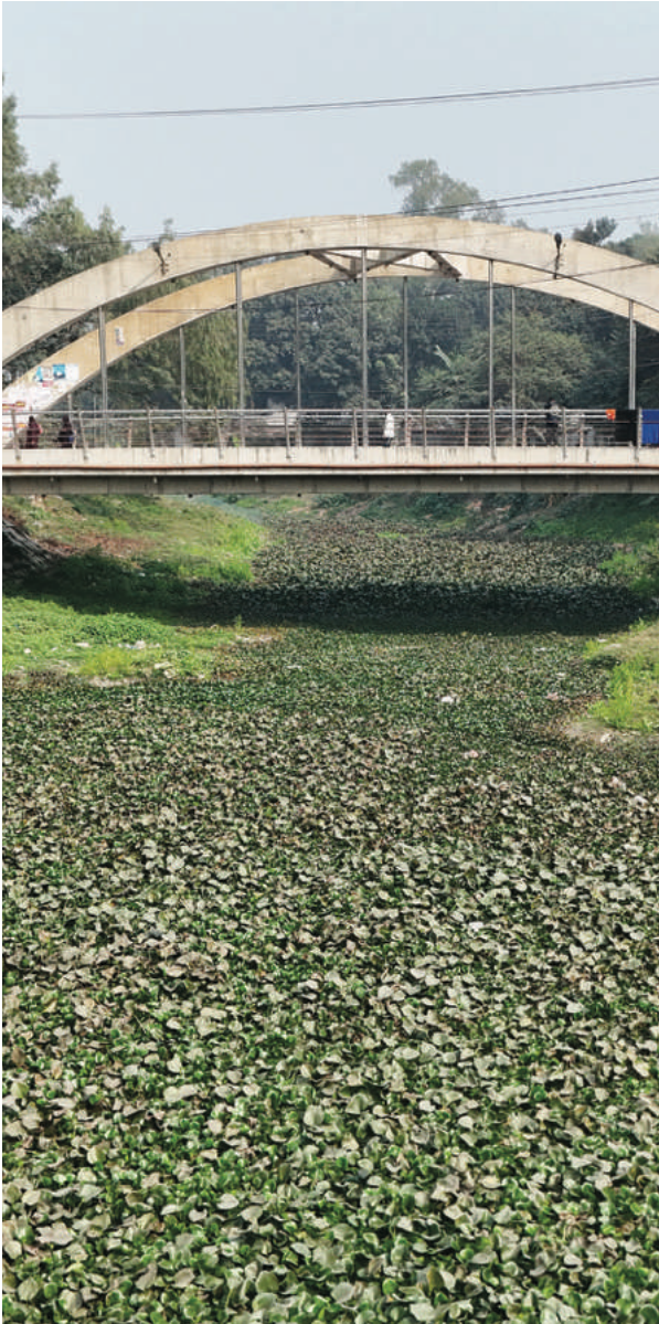
Photo 7: A view of the Katakhal Khal and a bridge across it
