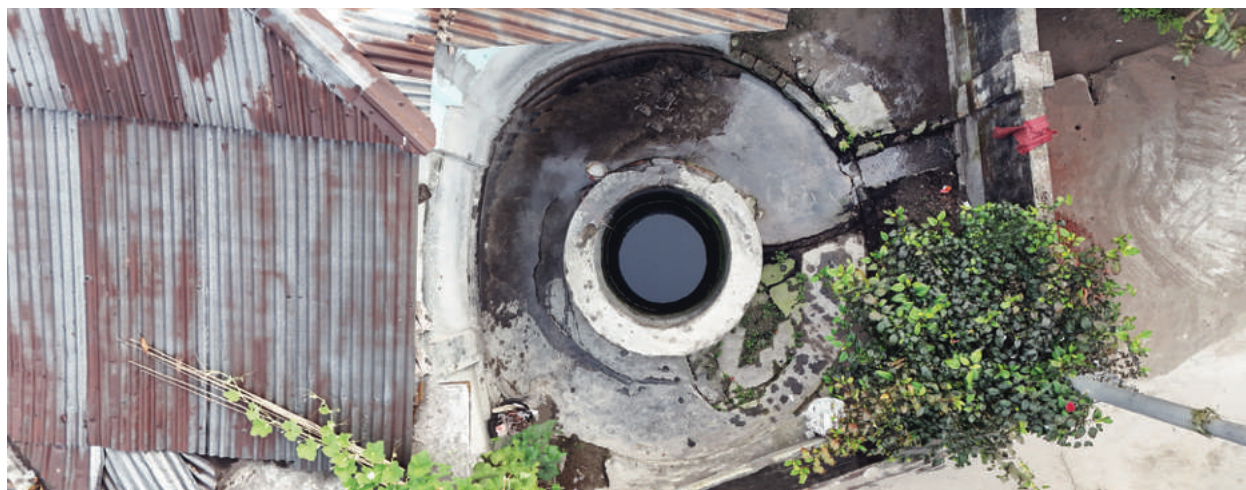
Photo 35: An aerial view of the dug Well, Nilphamari
