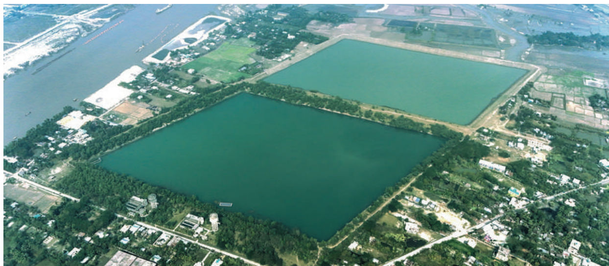
Photo 45: An aerial view of the Water Treatment Plant, Mongla
