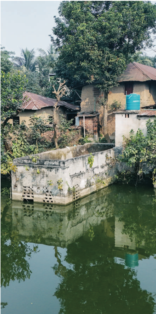
Photo 67: A view of the Bou Ghat within the Pond
