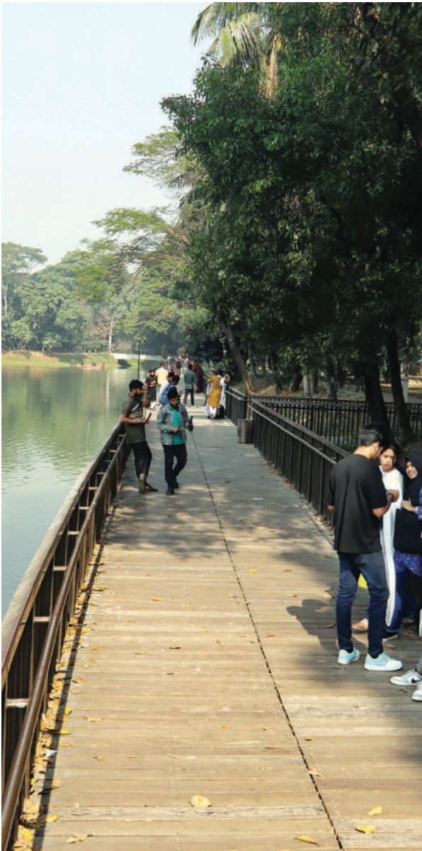
Photo 20: Recently built walkway along the lake's edge at Ramna Park
