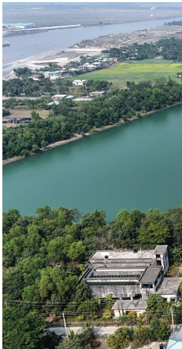
Photo 44: An aerial view of the Water Treatment Plant, Mongla
