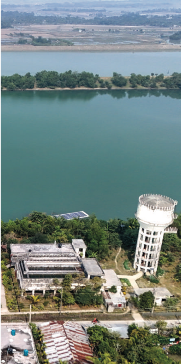
Photo 46: Two overhead water tanks located near the ponds
