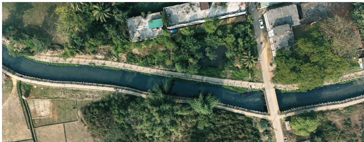
Photo 3 : Aerial View of Kudalichora Canal, Moulvibazar
