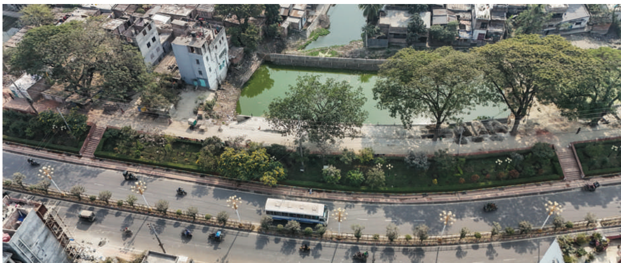
Photo 22: An aerial view of the Kolpona-Talaimari River embankment plantation
