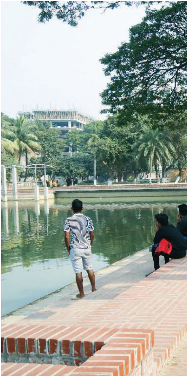
Photo 58: Steps and walkways constructed at the Haji Muhammad Mohsin Government High School Pond, Rajshahi
