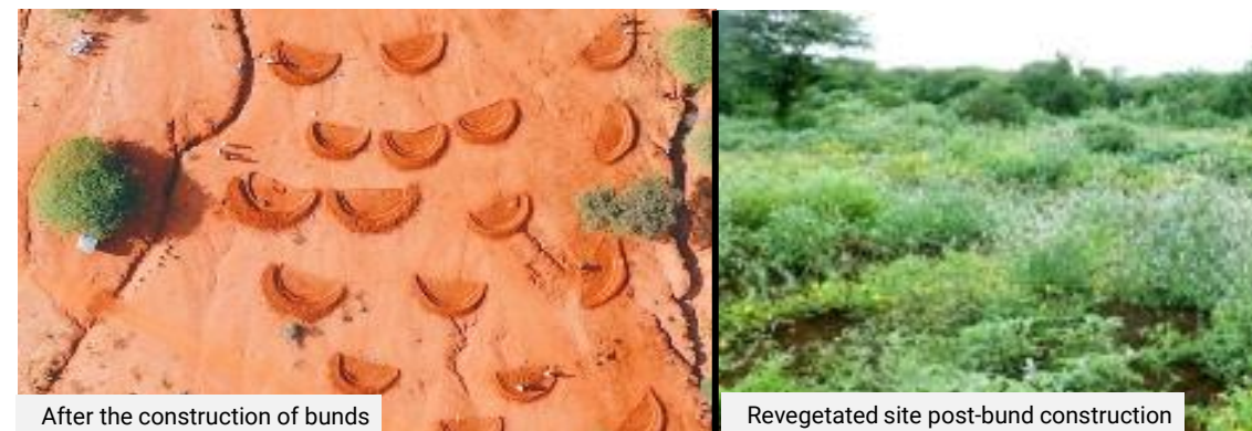
Figure 3 – A site after the construction of bunds and after revegetation (Source: https://ourworld.Justdigg.it.org/en/chapter/water-bunds )
