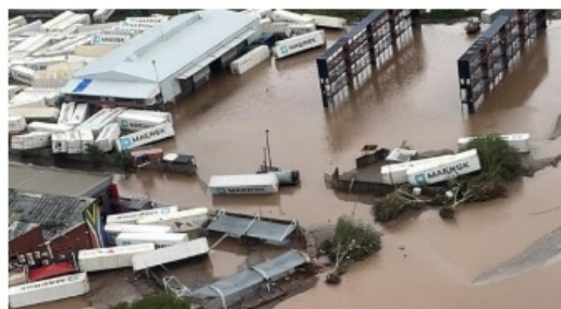
Port damage from flood (South Africa)
