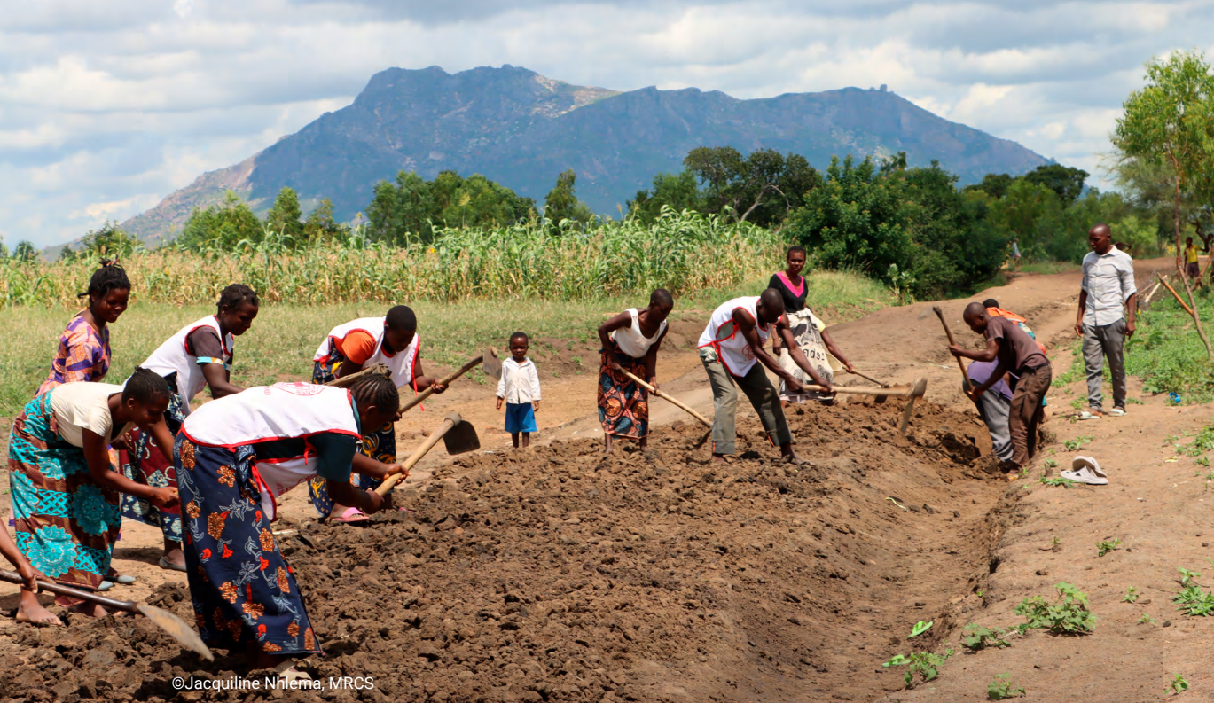
Members of Chitsanzo Group Cash Transfer in Malawi clear drainage for waterways.
