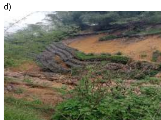
Figure 14. a) Stabilization of a gully head in Kinguari at Brazzaville, 32 b) Schema type of vegetated gabions, 33 and c) Stabilization of talus with gabions in Ngamakoso's road, 34 and d) gabions system failed installed in Talangai.
