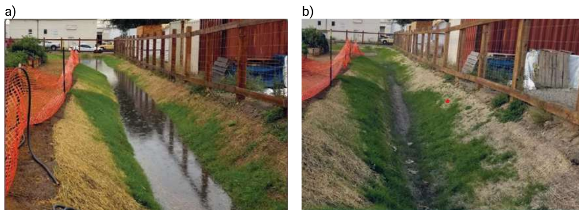
Figure 12. Infiltration swales a) during a rain event and b) within 6-12 hours after water is drained or infiltrated. 22
