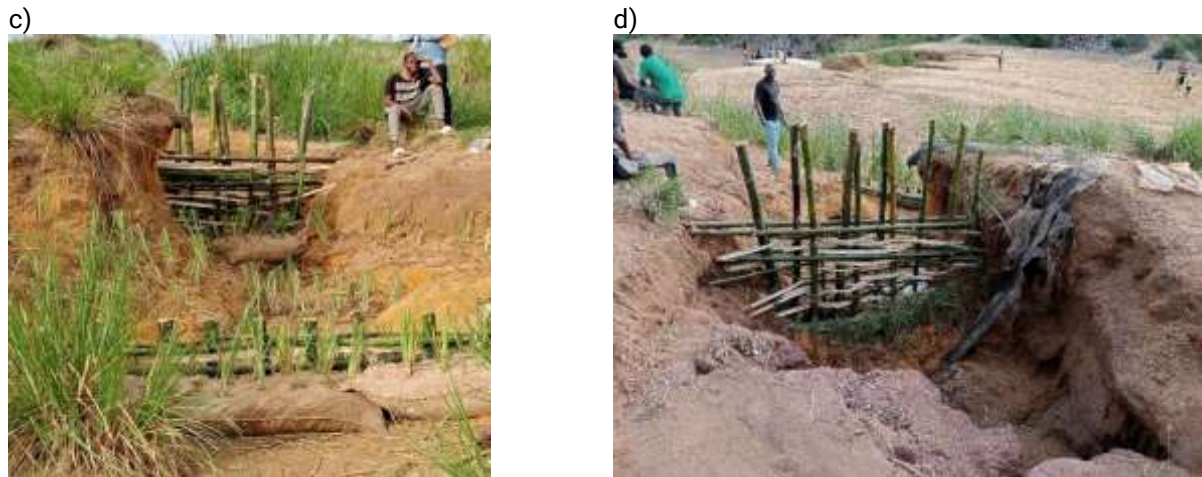
Figure 16. a) Wooden check dams after few rainy events, 50 and b) Gully control structures design details, 51 c) and d) Installation of wooden check dams by the community in Ngamakosso during training activities of this project, led by OCA in November 2025.
