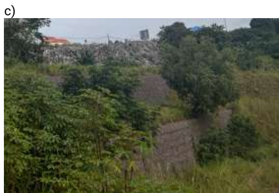
Figure 14. a) Stabilization of a gully head in Kinguari at Brazzaville, 32 b) Schema type of vegetated gabions, 33 and c) Stabilization of talus with gabions in Ngamakoso's road, 34 and d) gabions system failed installed in Talangai.
