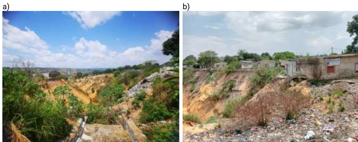
Figure 9. a) Single head cut gully with sandbags in cascade; and b) Abandoned houses in the Ngambio neighborhood.
