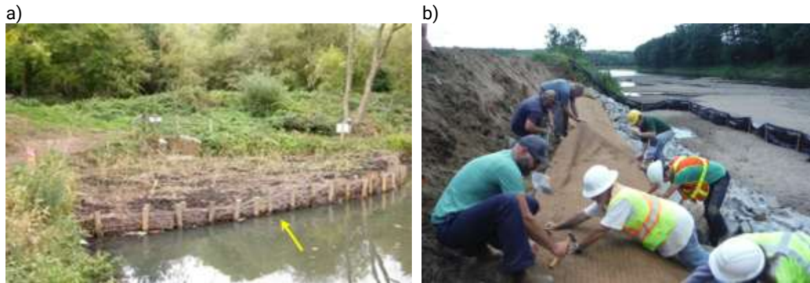
Figure 29. Live-fencing riverbank barrier (a) and organic soil stabilization mattress to be installed in combination with living stakes (b).
