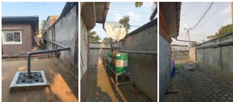
Figure 18. Infiltration pits installed on residential plots for runoff control near gully in Don Bosco.
