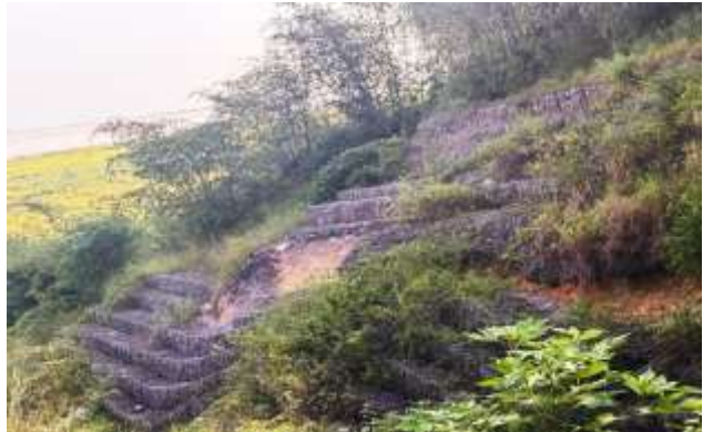
Figure 9. Vegetated gabions in Ngamakosso, Brazzaville
