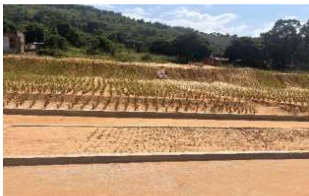
Figure 10. Planting of stabilizing vegetation at Ngamakosso Water Tower, Brazzaville
