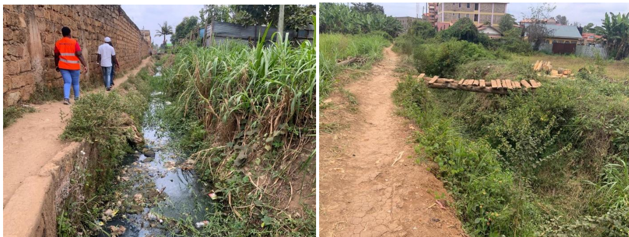
Figure 22: Open Sewer Channels in Maragua Town
