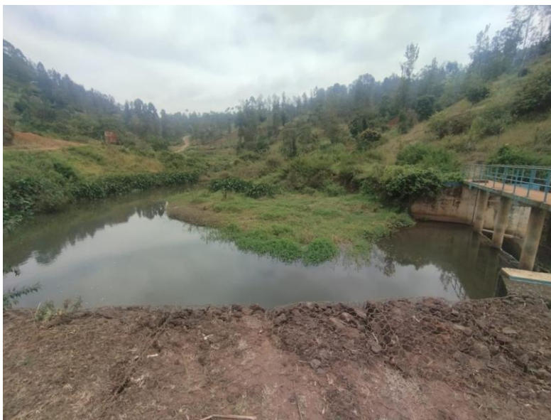
Figure 11: Shrinking Irate Intake reservoir capacity as a result of siltation caused by soil erosion
