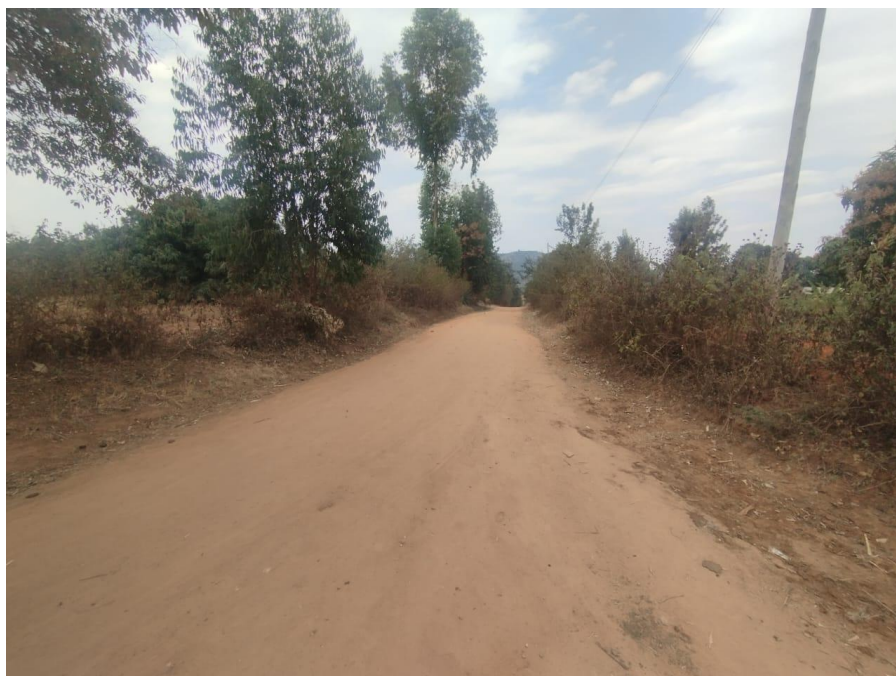
Figure 17: Road to Kwa Mukudi village where the main trunk line of the current water supply is located.
