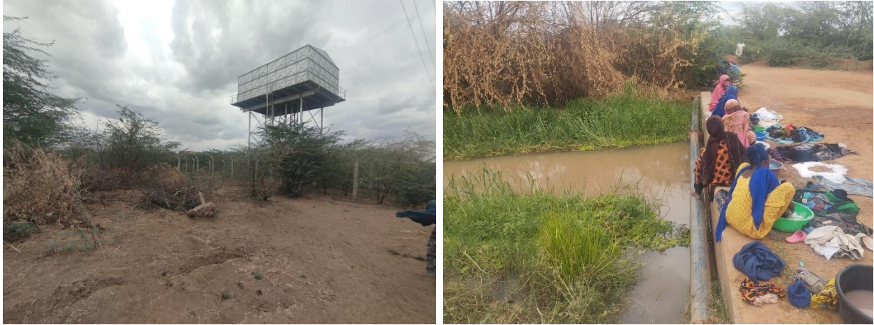
Figure 9: Bura Irrigation Scheme Storage Water Tank and Pipe Termination
