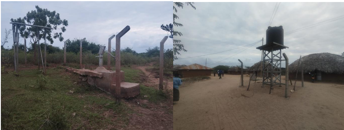
Figure 7: Mkomani Village Existing Raised Borehole Platform and Community Water Tank
