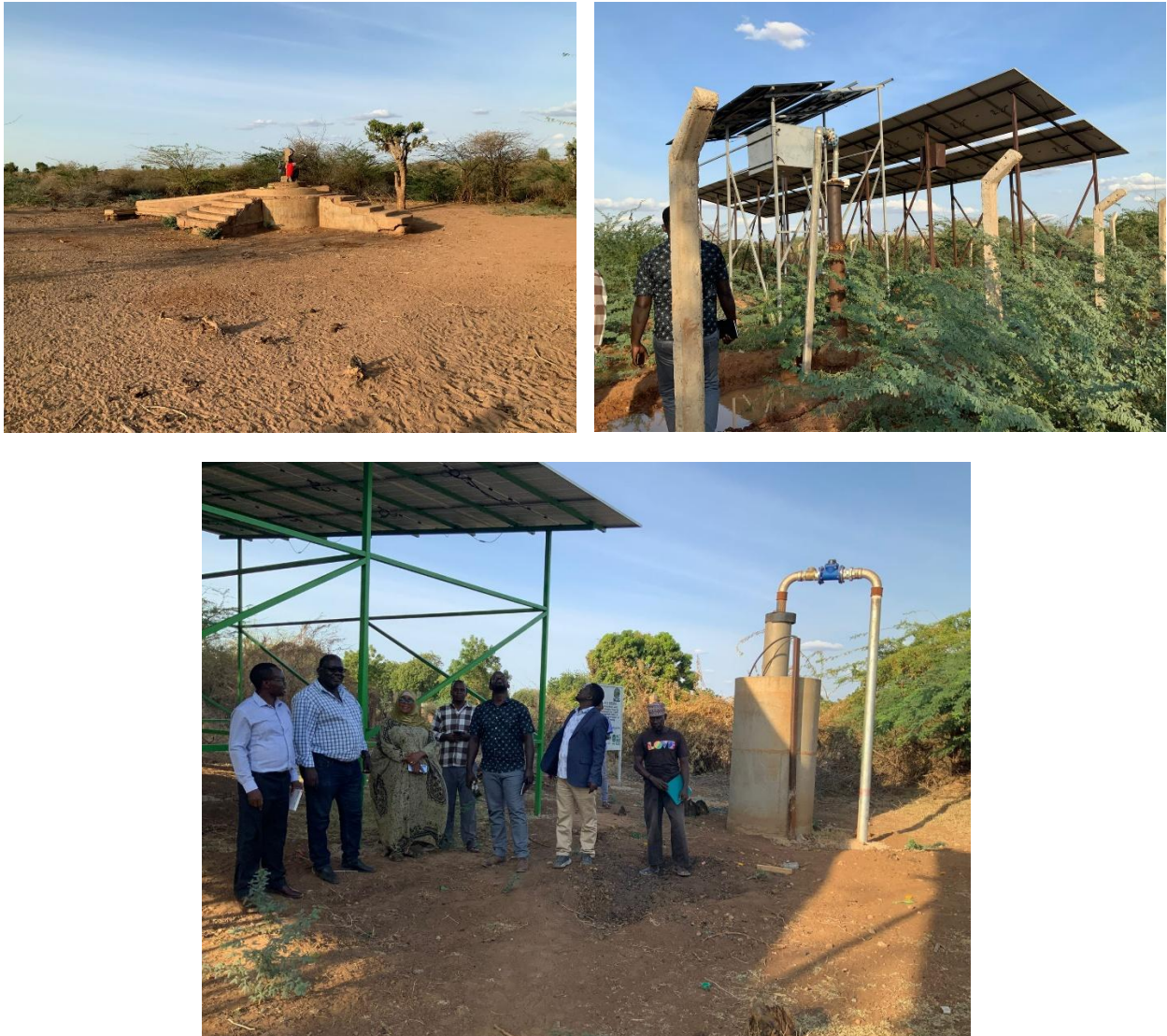
Figure 20: Operational, Solarized and Elevated borehole platforms in Madogo.
