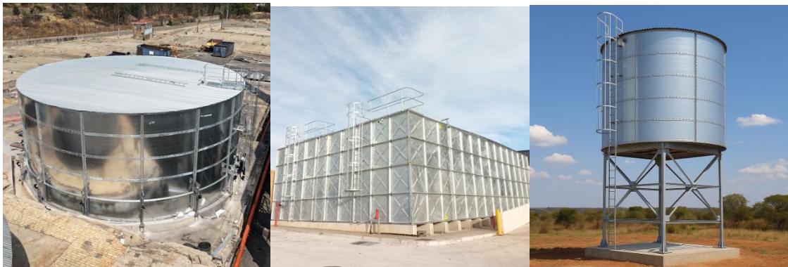
Figure 20: Example of modular water storage system (Photos from iWater company)
