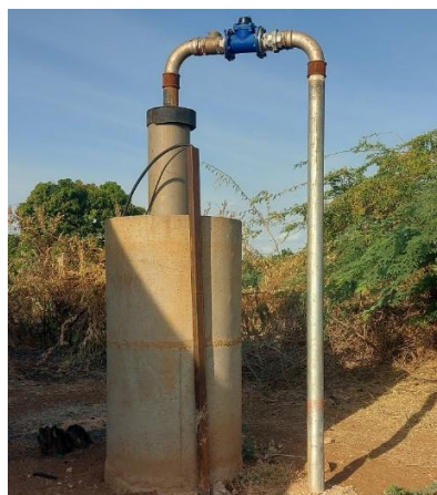
Figure 13: Borehole head with elevated concrete chamber
