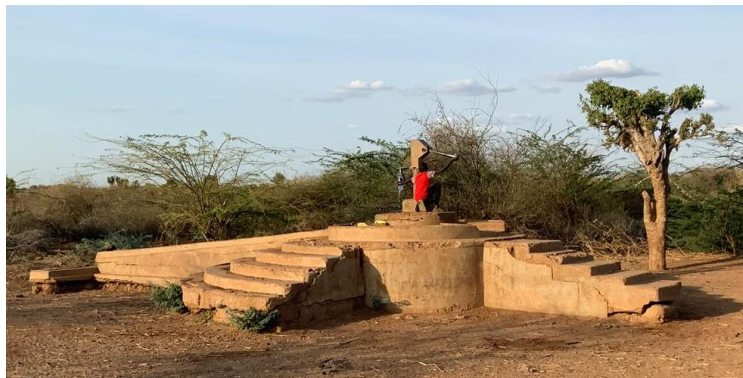
Figure 14: Elevated hand pump in Tana River
