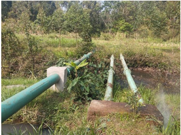
Figure 51: Relocated pipes running along River South Mathioya valley in Kiarathe with river crossing fitted with GI pipes from the joint chambers and also firmly anchored by concrete reinforced anchors.
