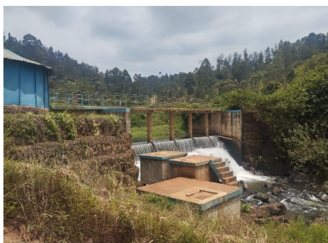
Figure 47: Irate Intake on River Irate in Gachocho area.
