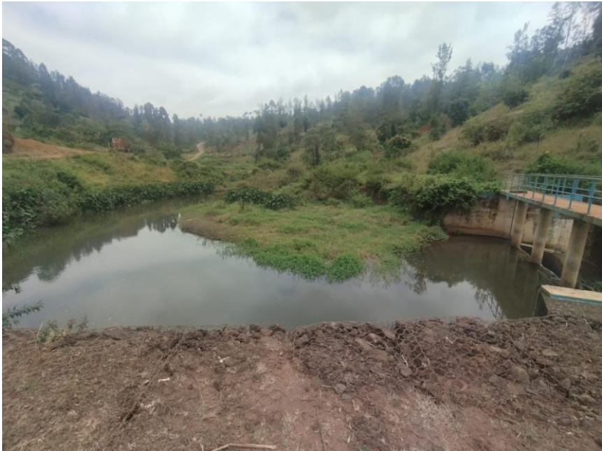
Figure 52: Shrinking Irate Intake reservoir capacity as a result of siltation caused by soil erosion
