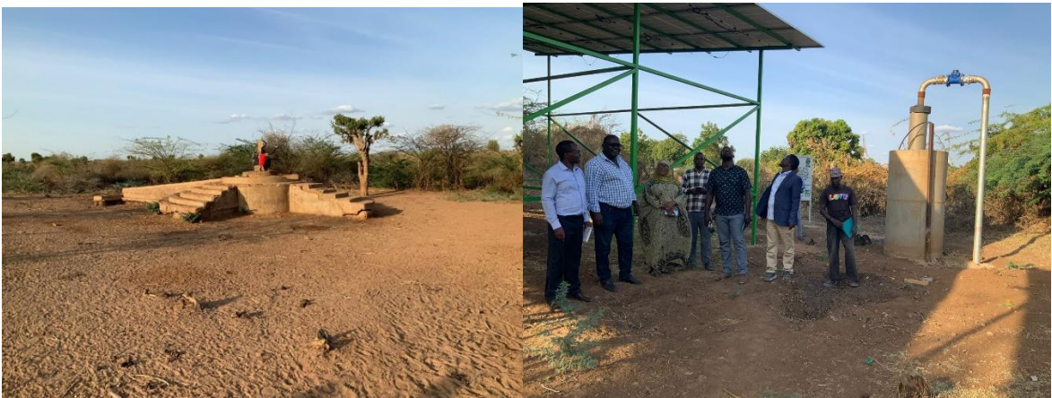
Figure 49: Elevated borehole platforms in Madogo
