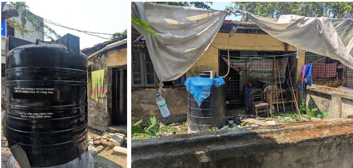
Figure 5.6: Existing rainwater harvesting system in Morrelganj
