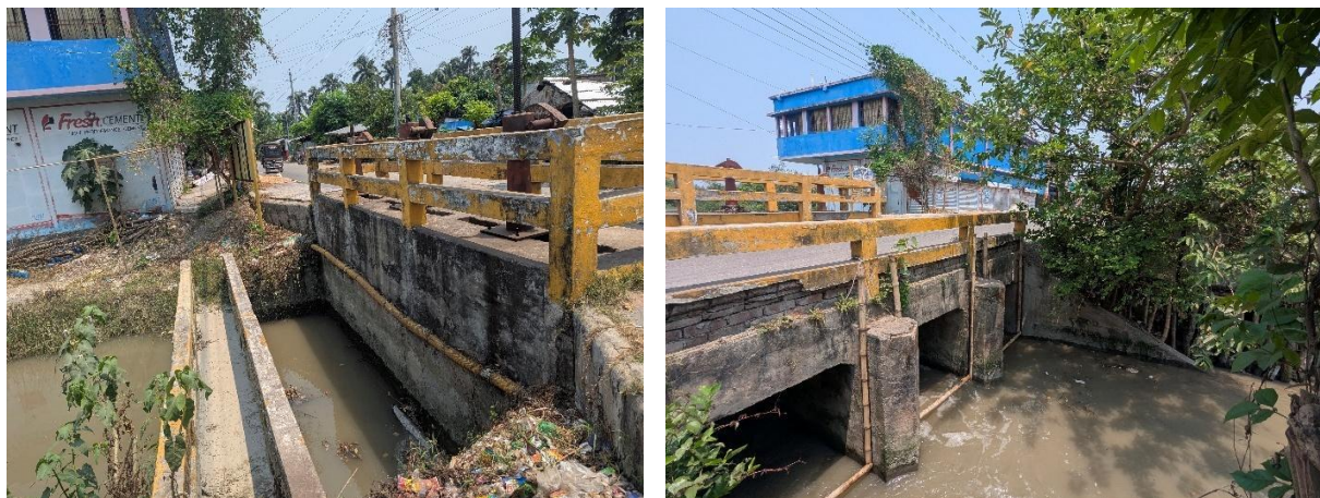
Figure 3.5: Partially functional three-vented sluice gate
