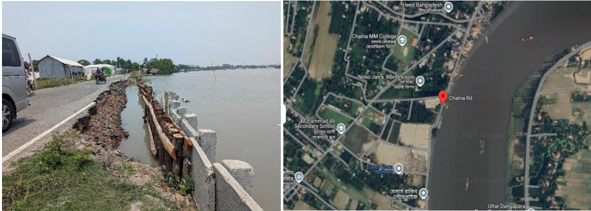
Figure 4.3: The erosion-prone Chalna road (left), and the dropped red pin shows the Google location of the site (right).
