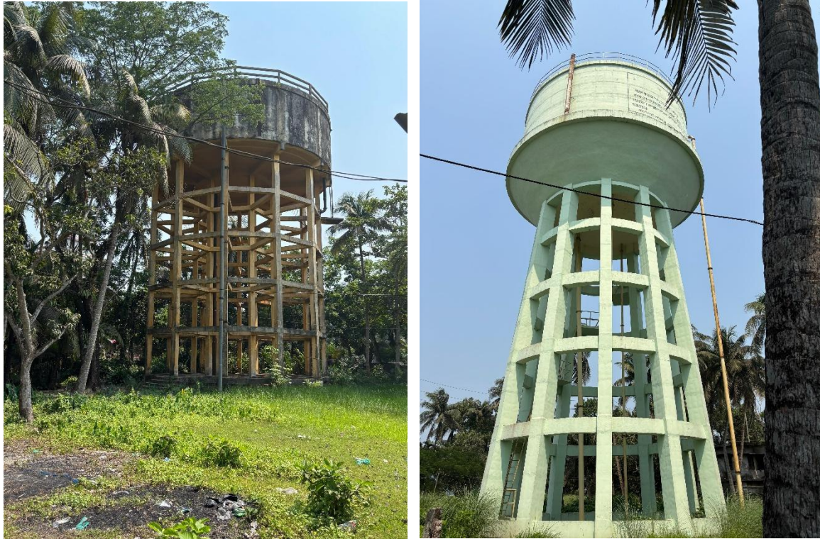
Figure 3.8: Ground water treatment plant (left) and surface water treatment plant (right)
