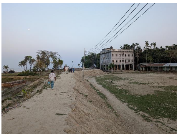
Figure 83: Road Infrastructure in Hatiya
