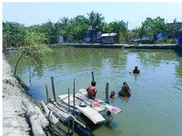
Figure 96: Water Infrastructure in Satkhira
