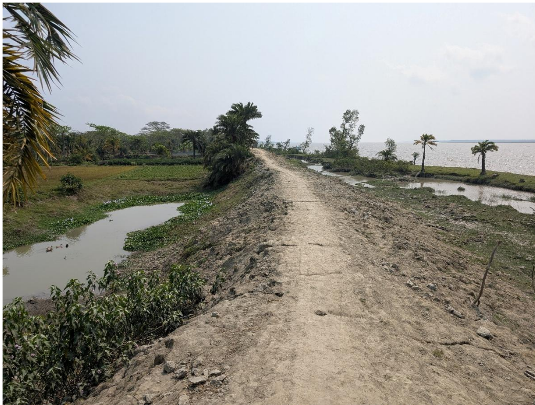
Figure 13: Road Infrastructure in Hatiya
