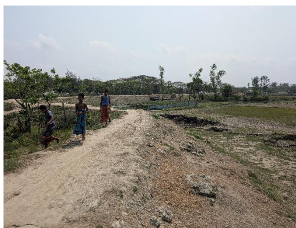
Figure 82: Road Infrastructure in Hatiya
