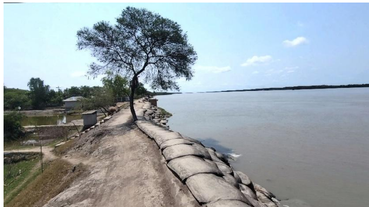
Figure 18: Coastal Road Infrastructure in Satkhira
