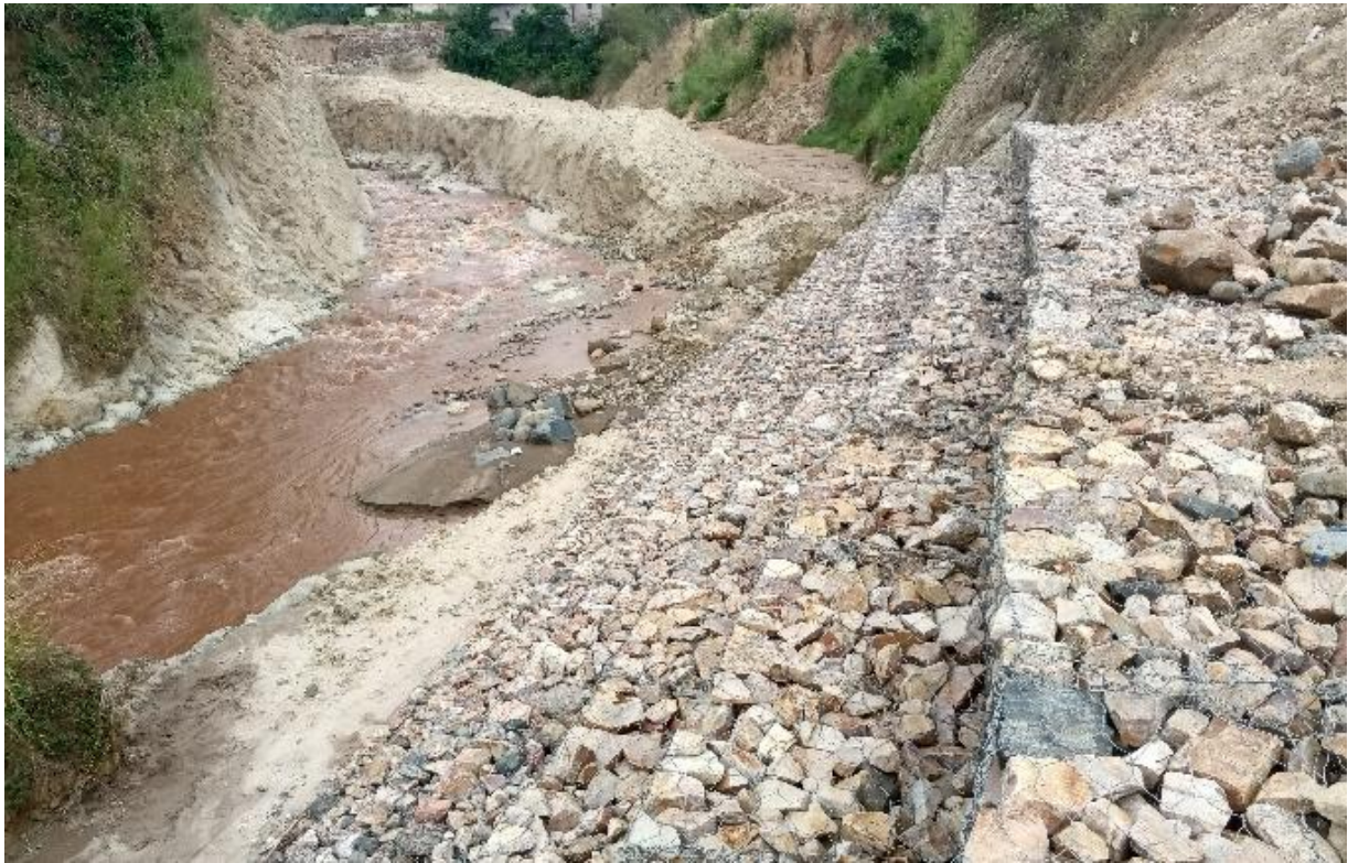
Figure 3. Gabions on riverbanks in Burundi xii
