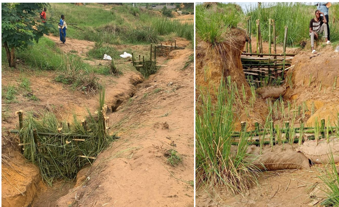
Figure 7. Vegetated check dams in Republic of the Congo
