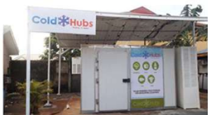
Solar-Powered Cold Storage for Milk
