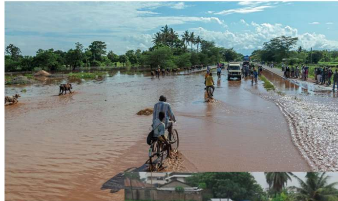
Flooding of roadway in Tanzania
